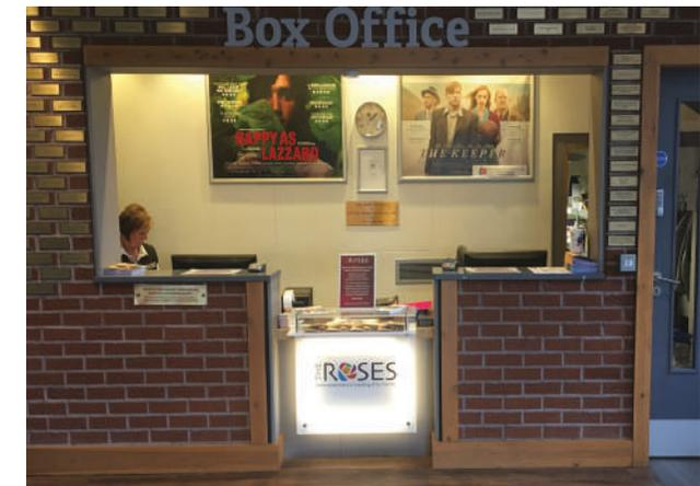
Figure 2: The lowered counter with large knee recesses allows wheelchair users to gain close access to the receptionist in this hotel
