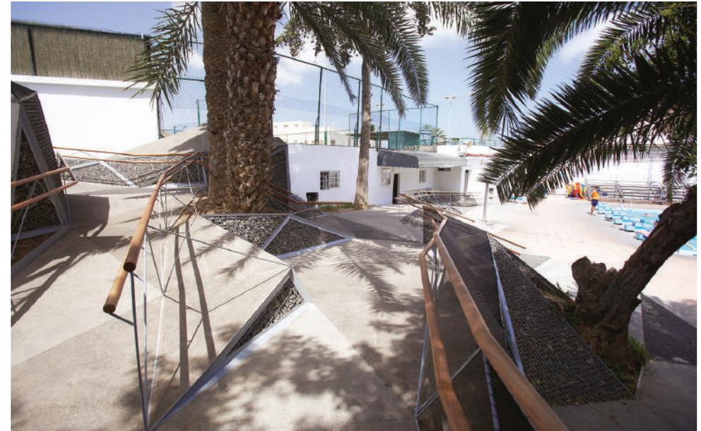
**Figure 1:** Planting areas have been integrated into this accessible ramp to provide visual interest and shade.
